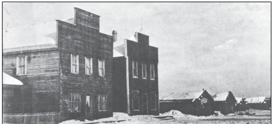
Whitecourt hamlet Main Street (north side, looking east): Harrop's Hotel, Old pool room (used for dances), Torgerson's Store, Torgerson's house, cache buildings. See map next page.
