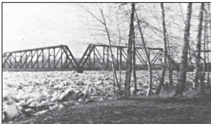
The ice piled to a point two feet below the McLeod Bridge in 1963 when the McLeod thawed before the Athabasca.
